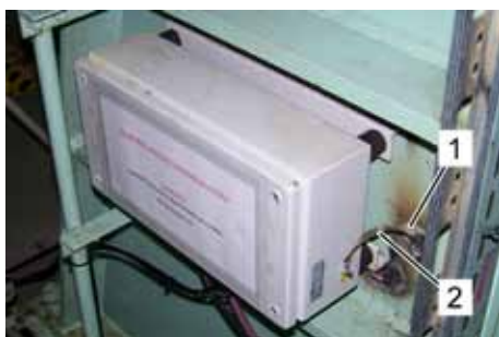
Fig. 64: Connecting earthing strap
