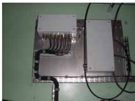
Fig. 65: Mounting bracket BLG00402 with the terminal box GHG002621... and one lineconverter box GHG002611...
