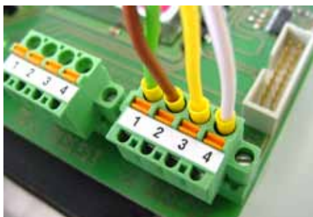
Fig. 73: Connecting the bus cables
