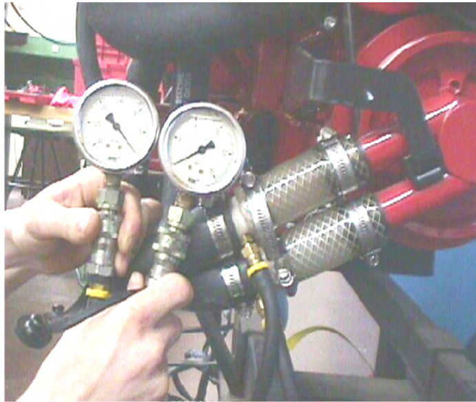
Figure 1 Installing Clear Hose at Raw Water Pump
